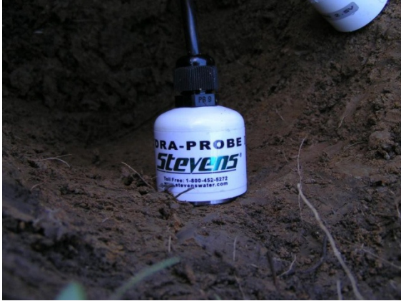
Figure 7. Installation of a Stevens Hydra Probe into native soil at a SNOTEL site [Bellingham 2].
